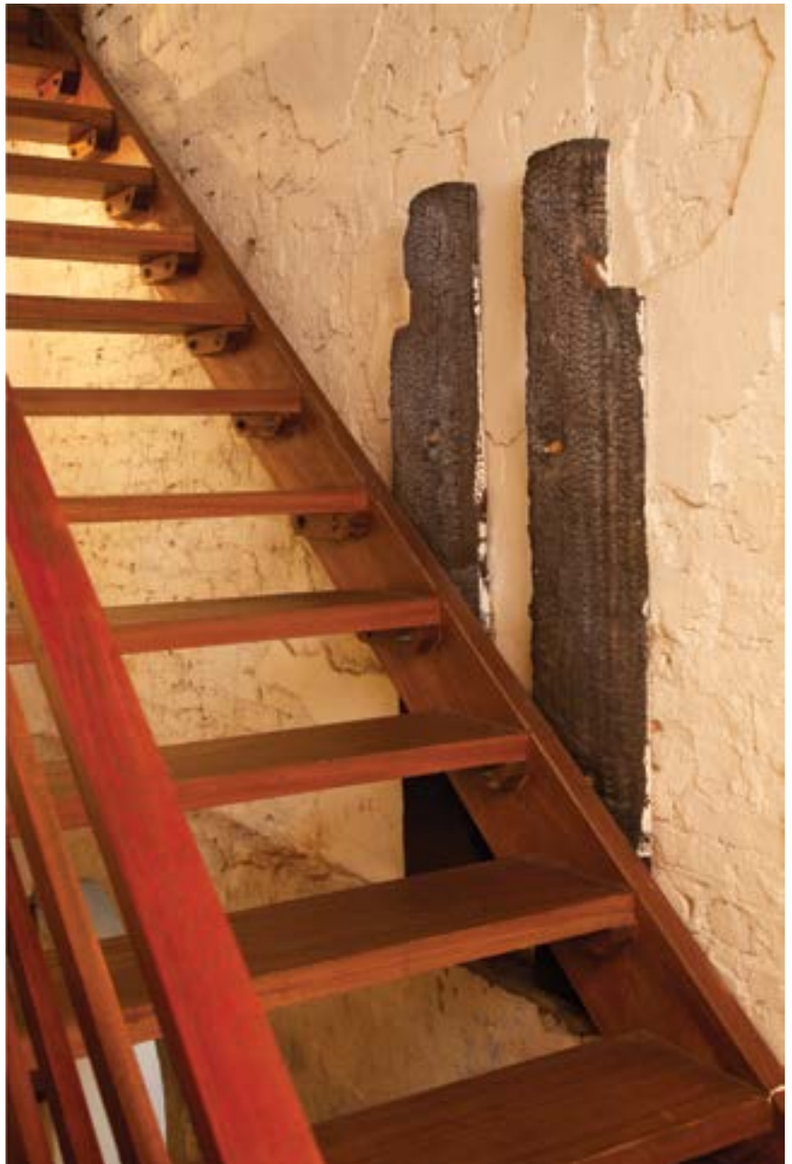
A flight of stairs bracketed off two charred timber posts that survived the fire. The charred timbers are meant to showcase the fact that timber burns slowly through a fire, enabling better predictability for any rescue operations.
