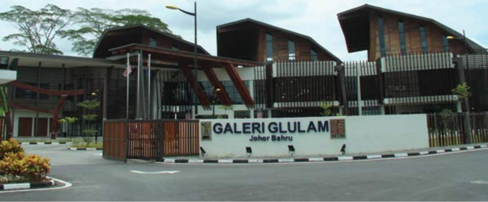
The building consists of three exhibition halls, formed by parallel portal frames and built using a combination of resak and keruing Glulam members. Photo credit: MTIB.
