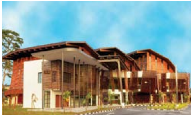
The building was designed as a three-portal frame with each consisting of eight glue-laminated sections connected by anchor plates and bonded in rods. Photo credit: MTIB.
